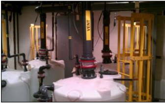
Davis Road PS Chemical Tank Replacement Project: is another example of a small project engineered and inspected in-house.
