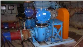
Brewerton WWTP Recycle Activated Sludge pump replacement: project was engineered and inspected in-house saving thousands of taxpayer dollars.
