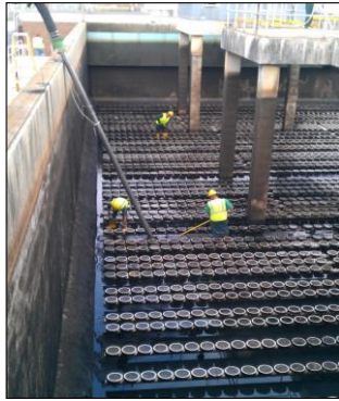
Metro WWTP Aeration Cleaning: Staff from Maintenance, Flow Control and Operations collaborated in an aeration tank cleaning project. Pictured here WEP personnel as they remove over 800 cubic yards of grit from the bottom of an aeration tank.
