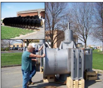
Metro WWTP Pump Replacement: 2011 brought about the conclusion of a multi-year project that replaced the influent pumping systems for the Metropolitan WWTP.
