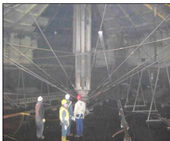
The Metro WWTP Digester Cleaning: project to clean and construct various improvements to sludge digestion system. Over 2,500 dry tons of material has already been removed from two of the four digesters and much needed repairs have been accomplished.
