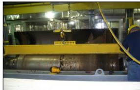
Pump Retro-fits: Metro Maintenance replaced 12 existing sand recirculation pumps connected to the Actiflo system. In a project done completely in-house, Maintenance personnel replaced the original pumps with a newer style pump requiring only a fraction of the cost to maintain. The cost of the new pumps will be recouped in less than two years with the county enjoying a yearly savings after that.
